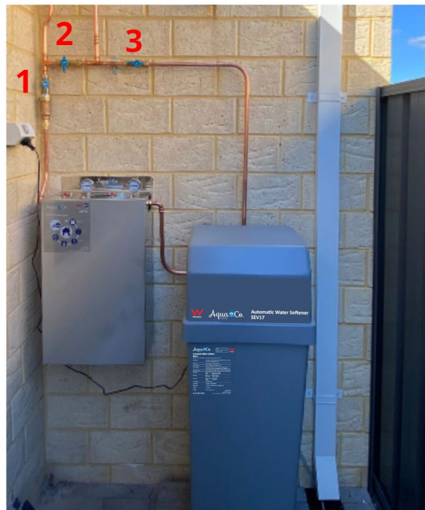
Valves 1 and 3 remain open. Valve 2 remain close.
